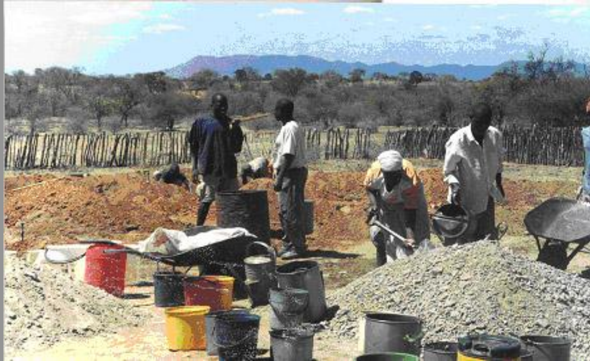
Picture 4: Mixing of concrete
